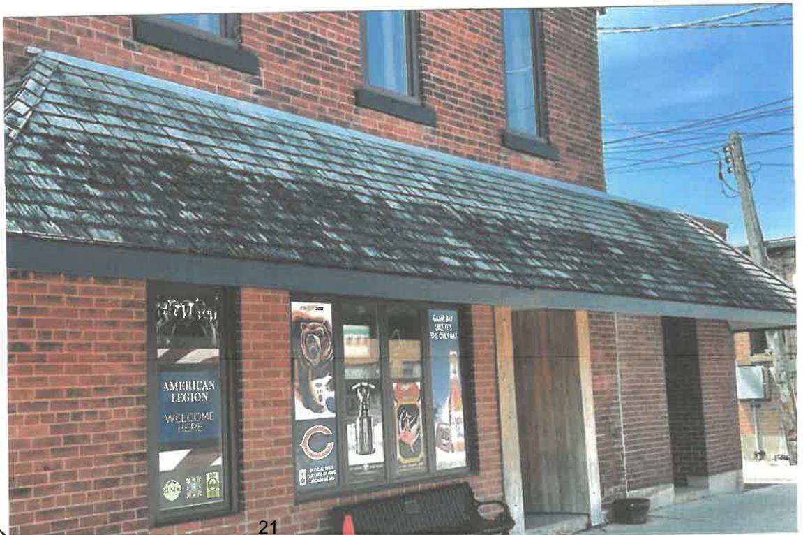
THE ENTIRE EAST SIDE WALL UNDER THE AWNING IS IN DESPERATE NEED OF TUCK POINTING. THIS WALL WILL BE REPAIRED.
